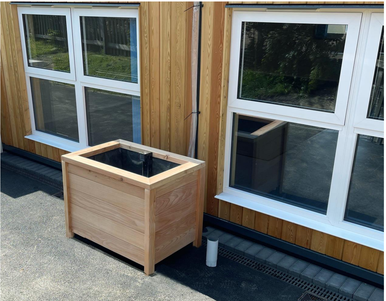
SuDS Planter in situ ready for connection
