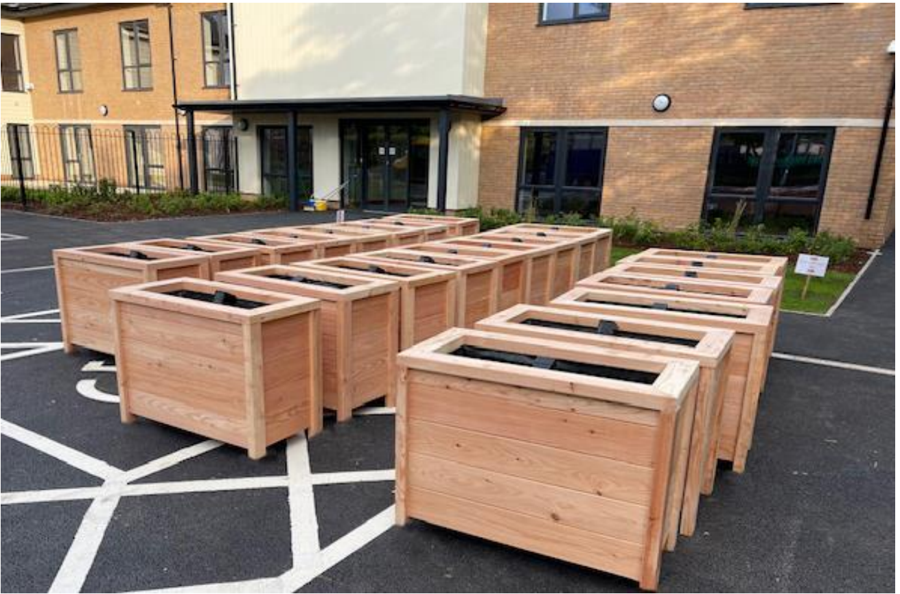
East of Eden SuDS Rain Garden Planters on site ready for installation
