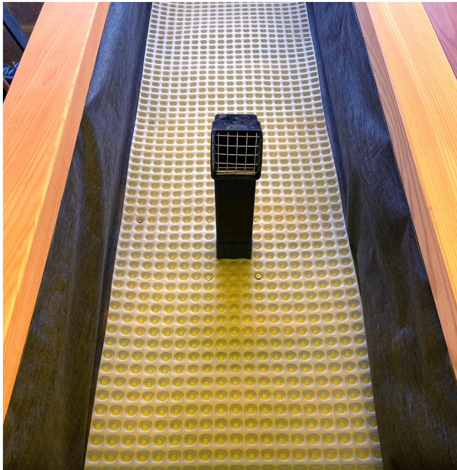
Geotextile layer with overflow ready for planting
